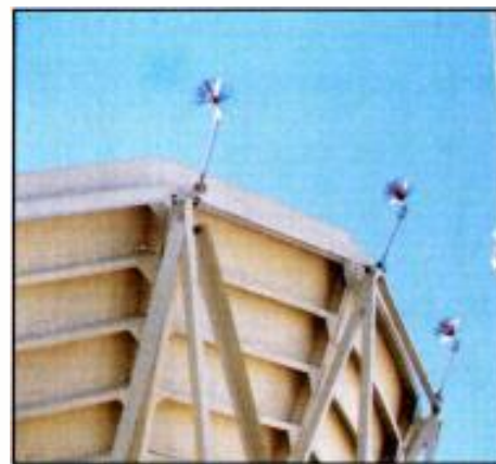
Although a satellite dish is not likely to be struck because of its rounded shape, it may still be vulnerable due to secondary effects of the ground charge rushing to a nearby strike. The dissipation array helps bleed off the accumulated ground charge.
